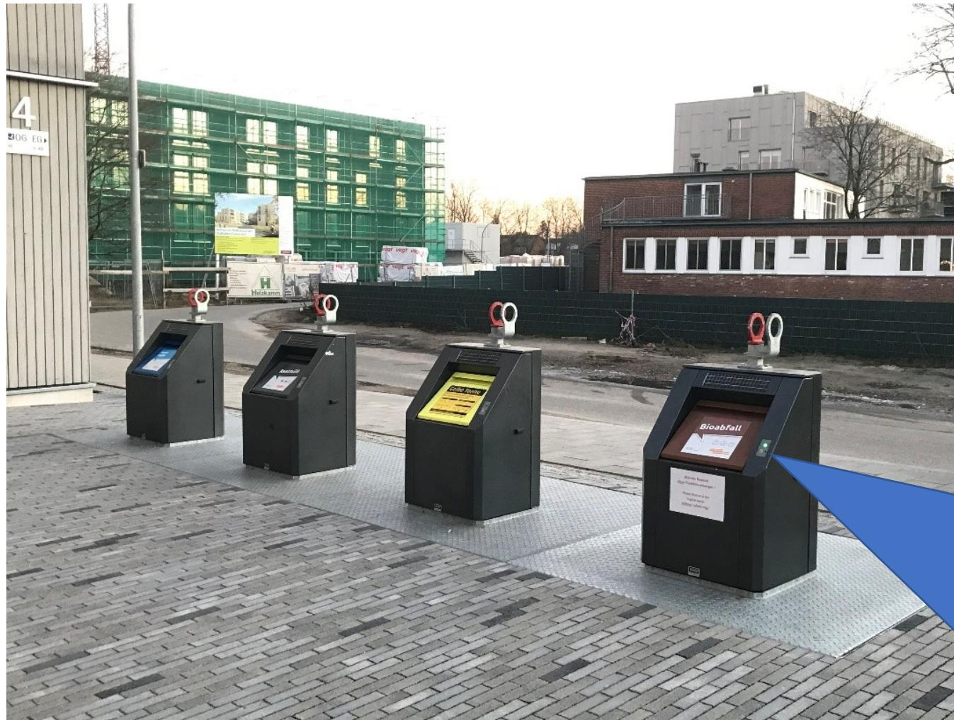
An underground container is equipped with an RFID unit. The built-in electronics first check whether the transponder is "permitted", if it is released, the lid can be opened, the waste falls into the underground container and the usage is stored with an RFID number, date, and time.
